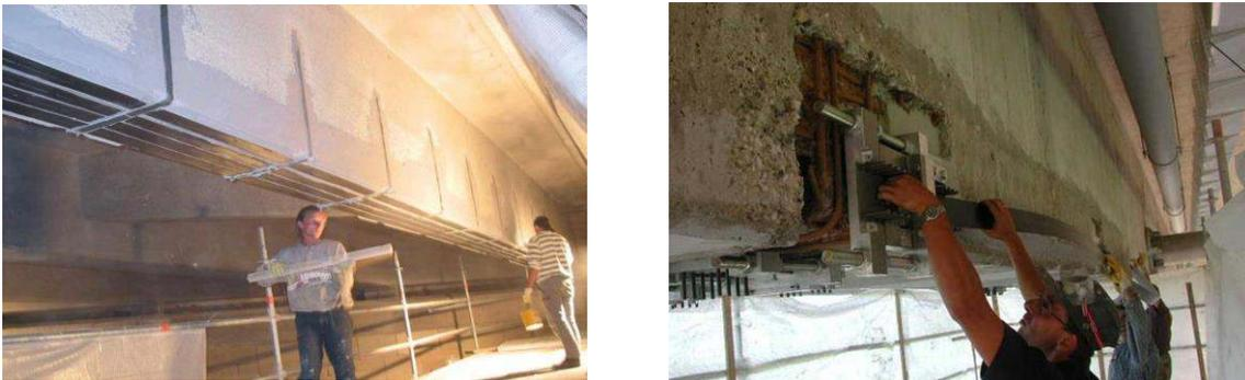
Figure 1: Two examples of the application of CFRP-strips to a bridge construction (HP-TL); left: Retrofitting by adhesively bonded slack CFRP-strips; right: Post-strengthening using a pre-stressing system
